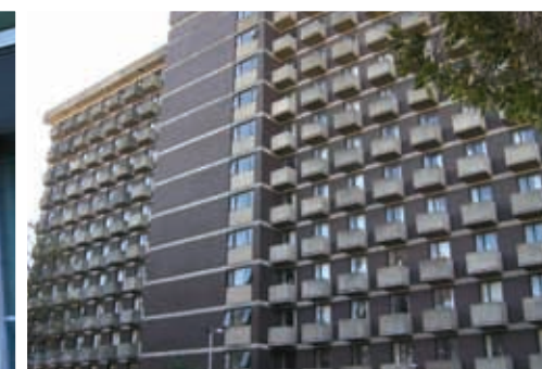
Vera Adderley Building, Randwick Closed 2009
